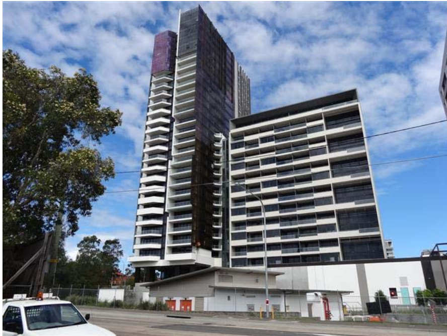
Figure 16: Adjacent development to the south within Victoria Square (20 Gadigal Avenue)
