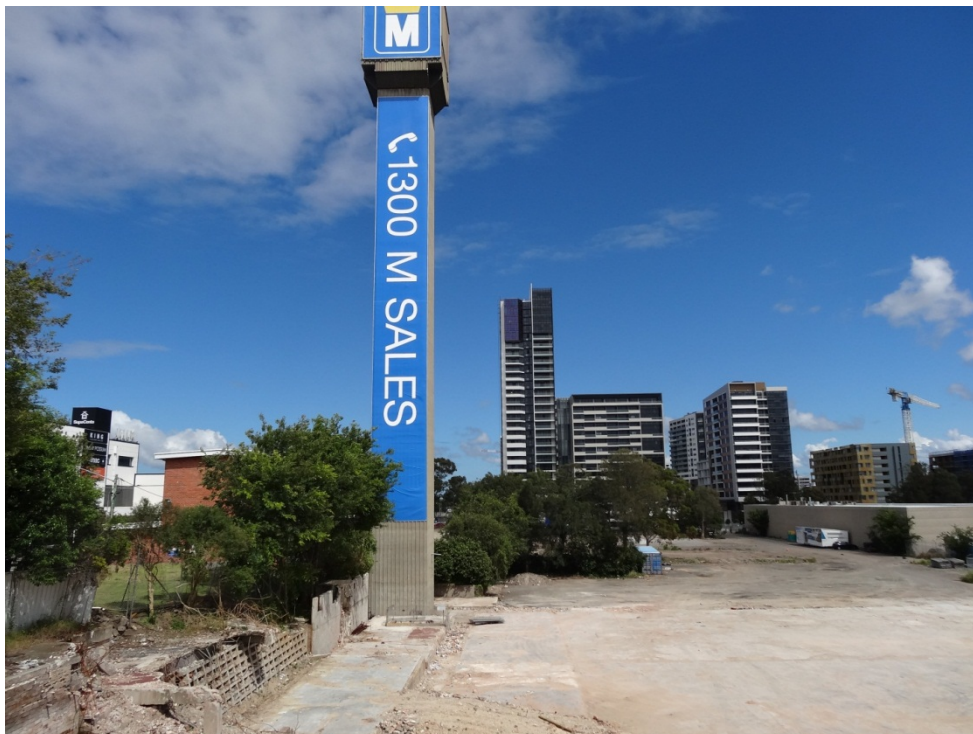
Figure 4: View of lift tower looking south from Shell service station
